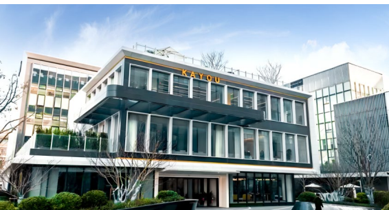
Application in office building projects
